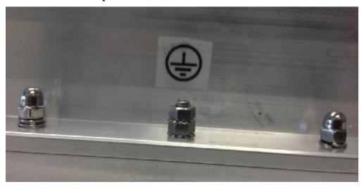
Figure 5-1 – 9502 Protective Earth Grounding
